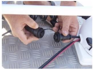
Note: Cut the existing control cable as close as possible to the Minkota's main mother board.....you need every mm to terminate this cable to the new male in line 7 pole plug from RS Components. The new female free socket is terminated to the foot controller cable & the pin outs marry as indicated above. All individual conductors require soldering at each end to
